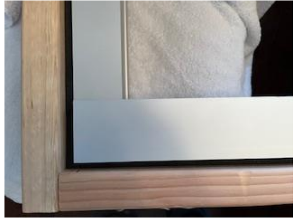
Jamb and sill flashing joint
